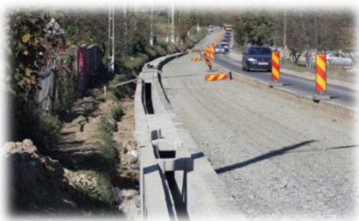
Figure 7. Roadway culvert
