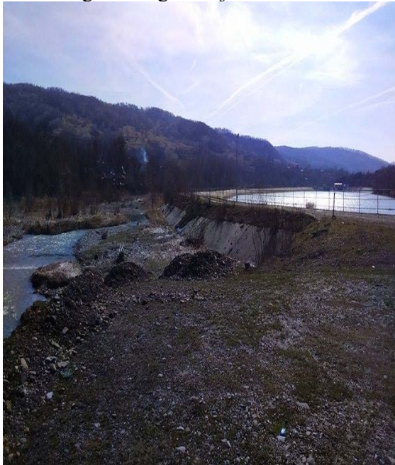
Figure 2. Deep erosions on longitudinal dike of the polder
