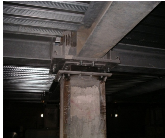
Figure 5. Example of application of base isolation method
